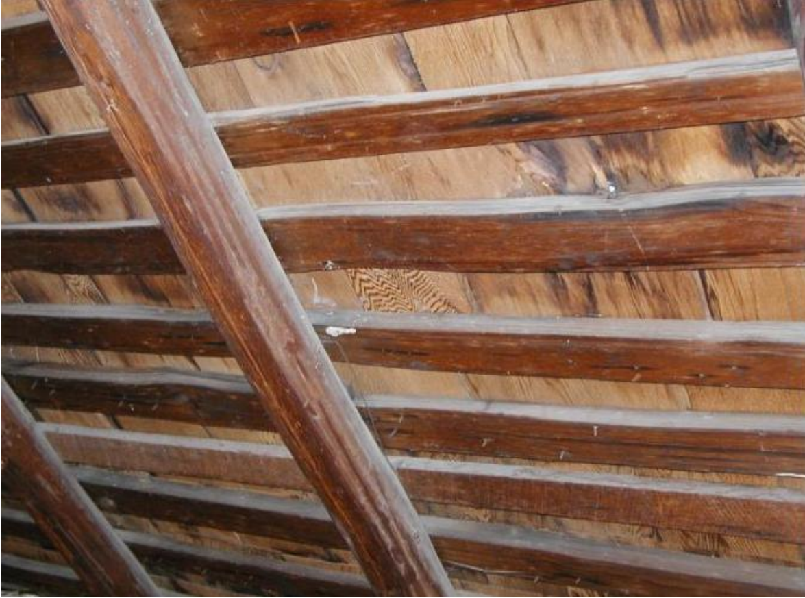
Attic joists, strapping and cedar shingles fastened with square nails
