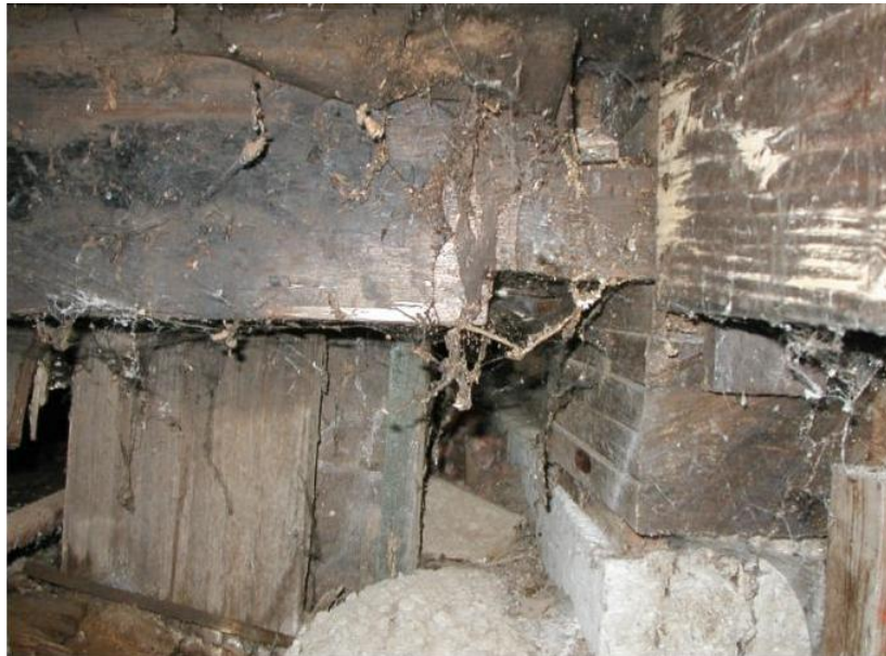
Wood structure in crawl space
