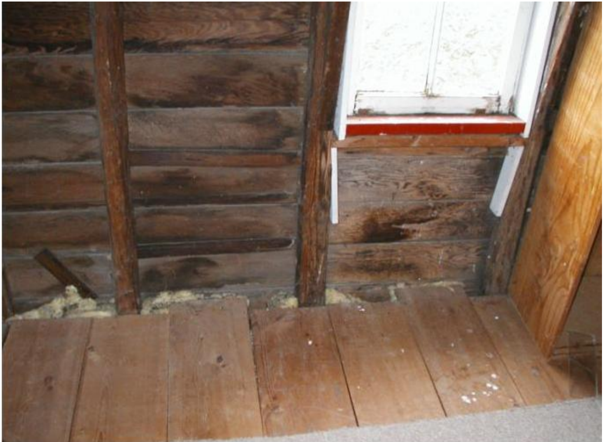
Balloon framing in attic
