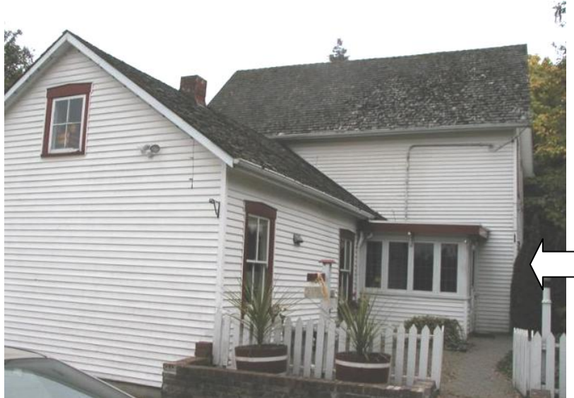
Porch and west façade of first addition, original house behind.
