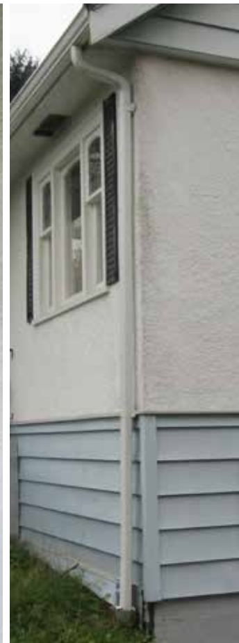
Gutter and downspout
