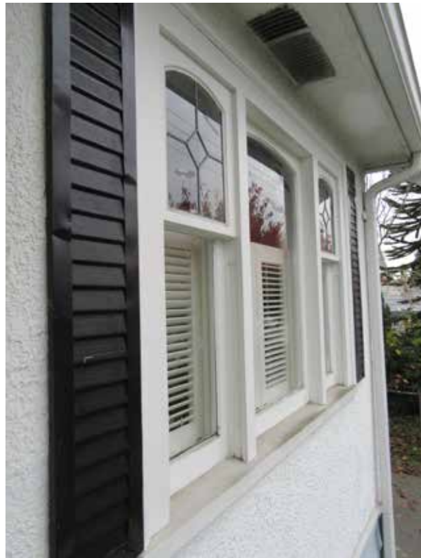
Top & Bottom: Original tripartite window with upper sashes featuring leaded glass
