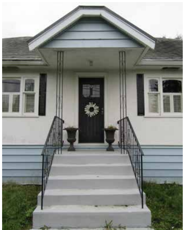
Top: Northwest view of porch; Bottom: Direct view of porch
