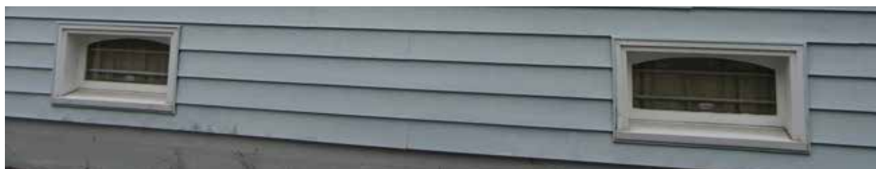
Top & Bottom: Original basement windows with wood sashes and arched headers
