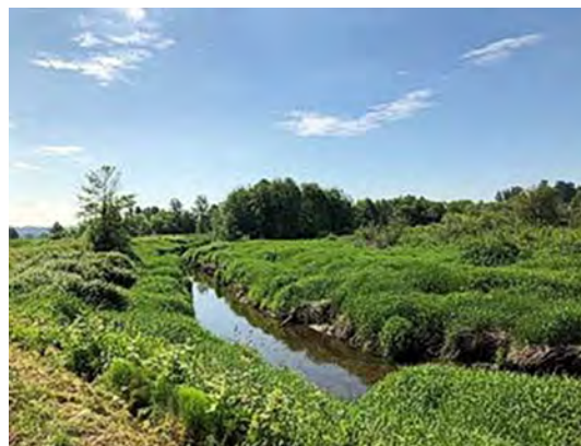
Drainage Infrastructure within the flood plain
