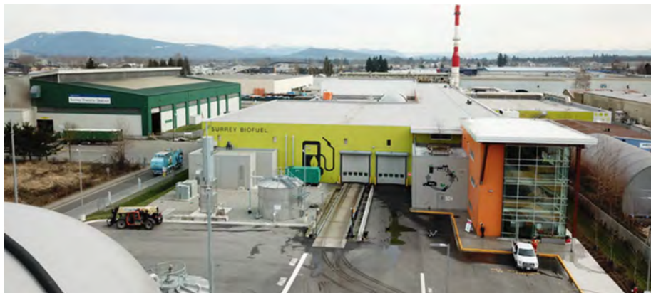
Surrey Biofuel Facility, City of Surrey
