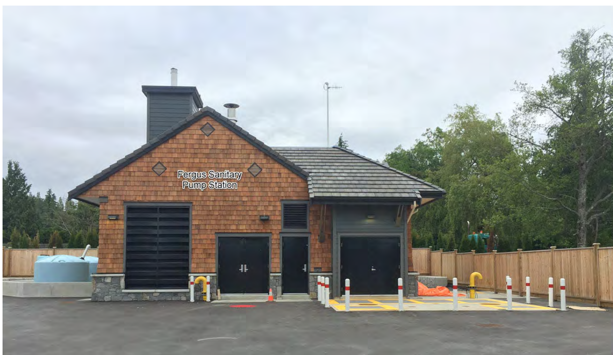
Fergus Sanitary Pump Station
