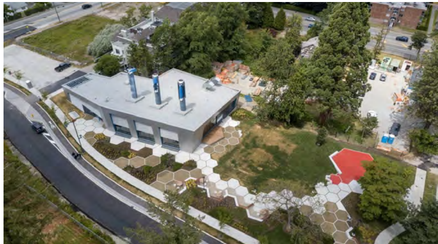
Surrey City Energy’s West Village Energy Plant
