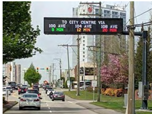
Surrey's Advanced Traveller Information System ("ATIS") is designed to improve the mobility, safety, and user experience.
