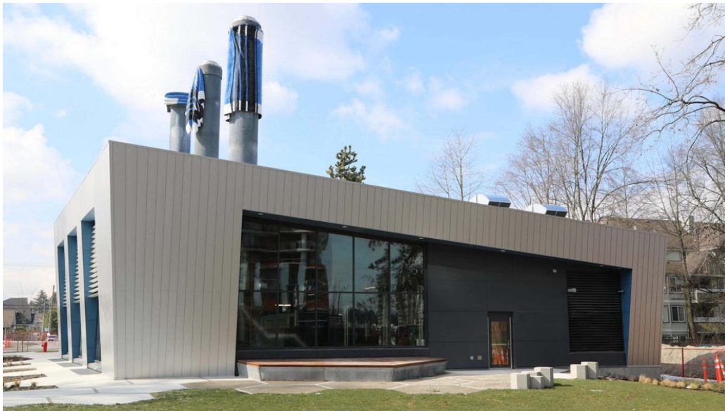
Exterior of District Energy Building
