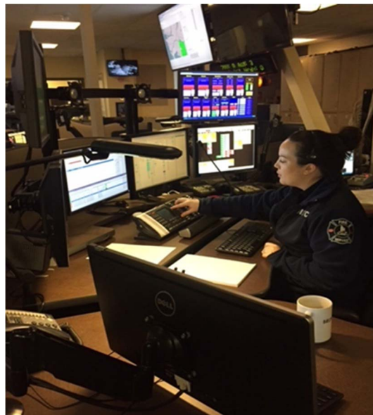
Surrey Fire Regional Dispatch Centre
