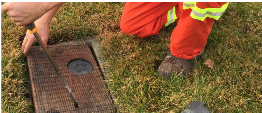
Water operator inspecting a meter chamber
