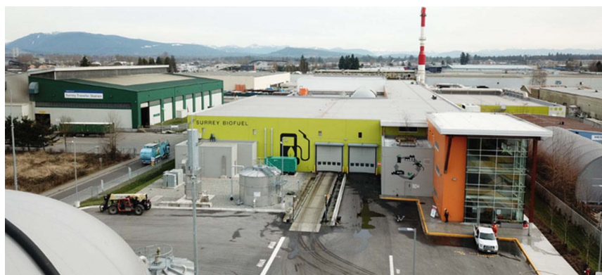
Surrey Biofuel Facility, City of Surrey
