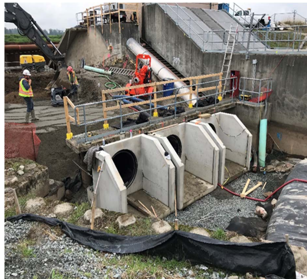
Flood Box Replacement at Fry's Corner Pump Station.
