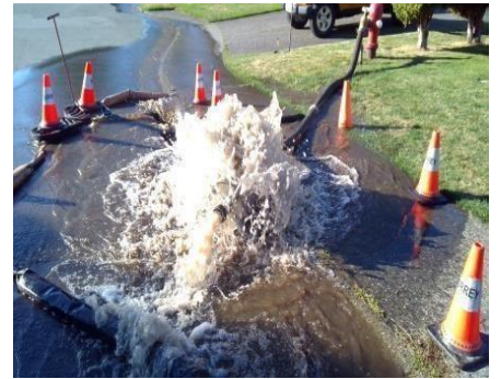
Typical set-up for water main flushing
