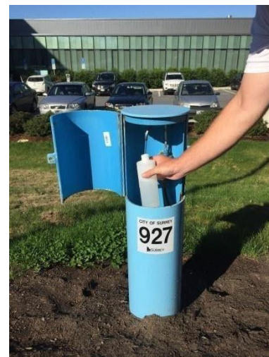
Water Sampling Station at 148 Street
