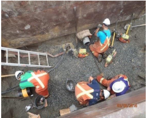
Water Main Tie in at 145 St & 109 Ave
