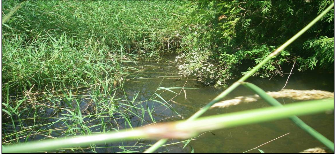
Photo 14. Looking upstream (west) towards the culvert draining “Stream B” under 168 th Street. Juvenile salmonids were observed in the pool habitat unit shown.
