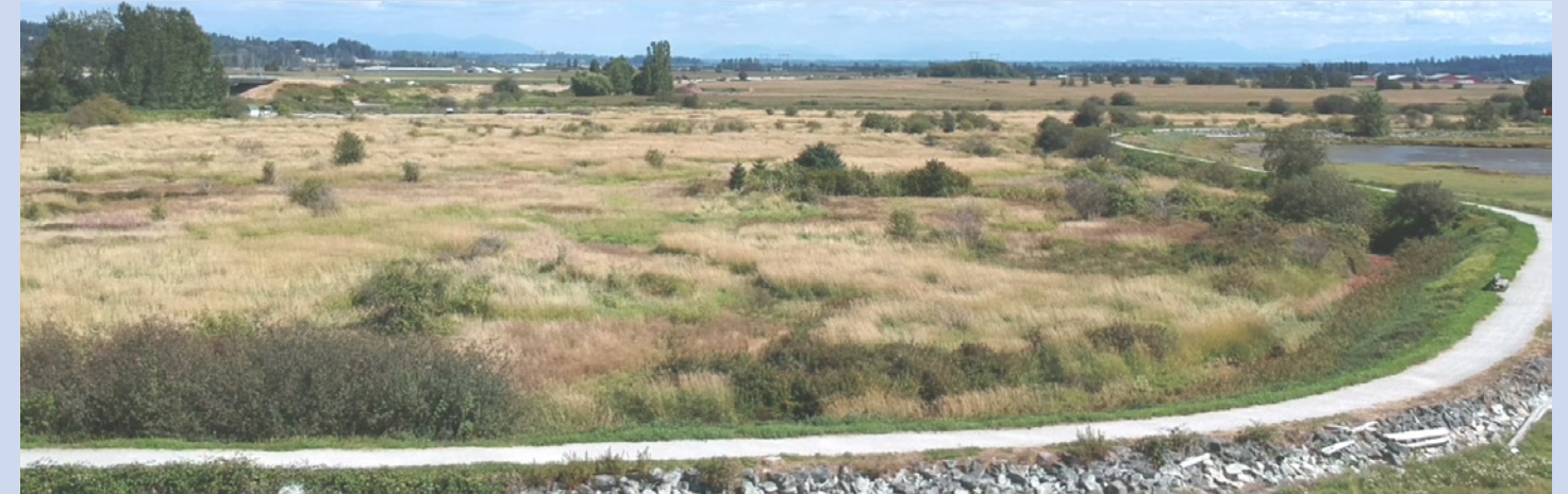
Maintain flood infrastructure: raised dykes
