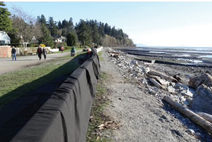
Temporary concrete barriers put up after March 10th, 2016 storm damage.
