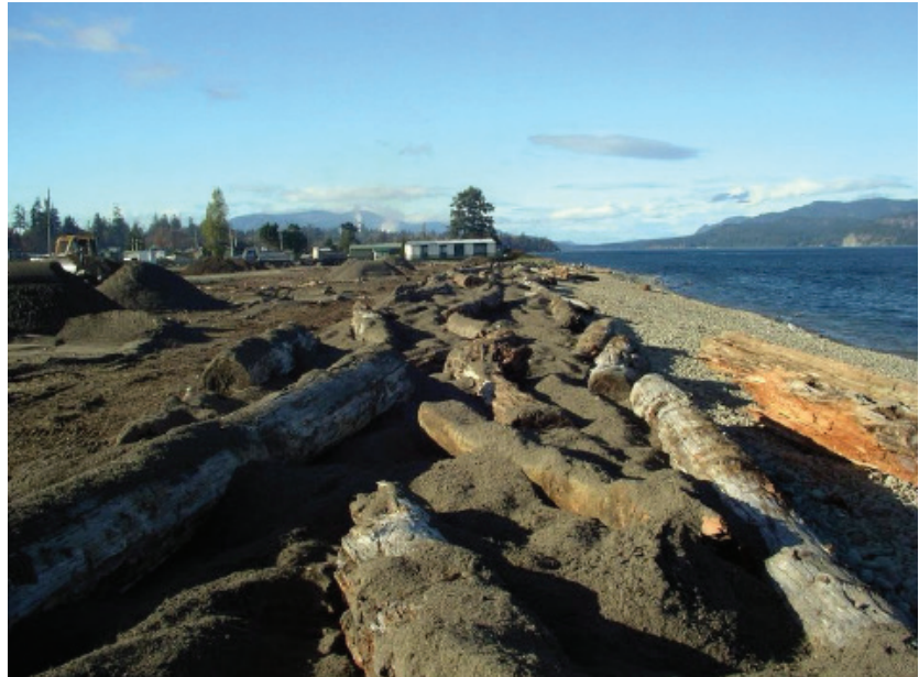
Example of a soft shore approach, using logs and natural materials to stabilize the beach. Photo by: Pat Harrison
