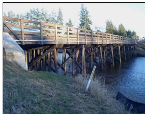
Existing Nicomekl Bridge
