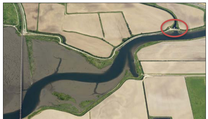
Mouth of the Serpentine River with Colebrook Drainage Pump Station (view from south)
