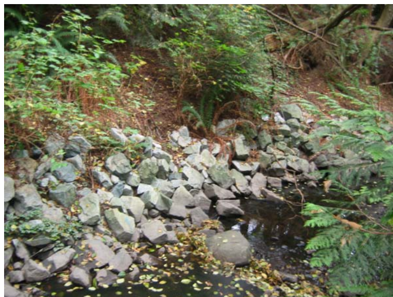
Photo 4: Example of Area of Terrace Instability with Stabilization Works
