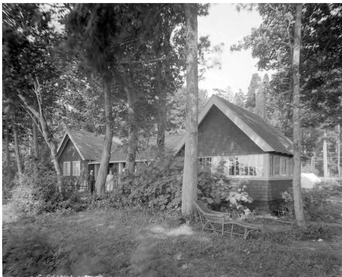
Mayor Gale's Summer Cottage at Crescent Beach, 1920, CVA A16948
