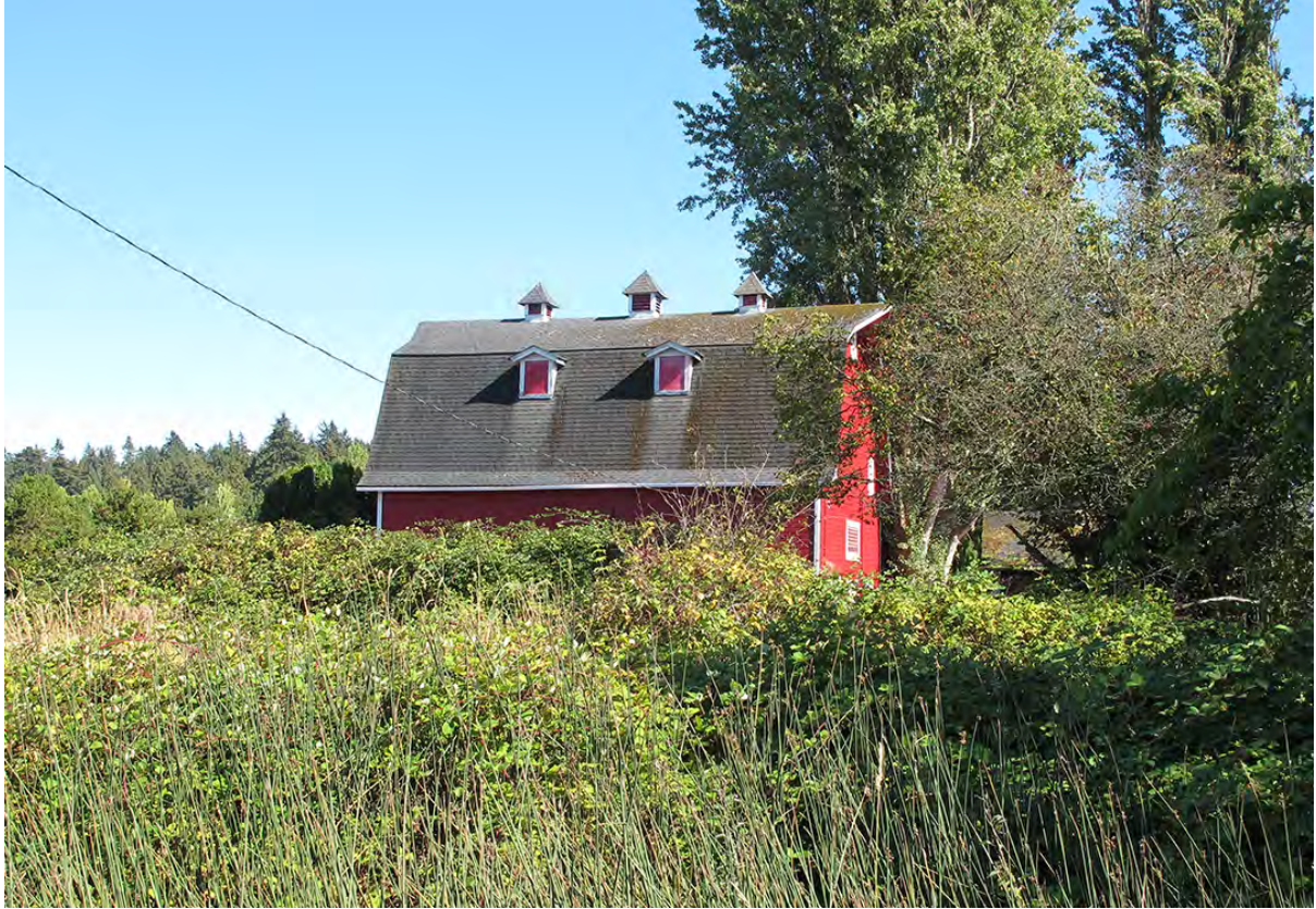
Barn, 12335 Sullivan Street
