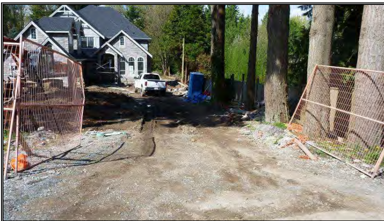
Development in progress at 10521 - 127 th Street.
