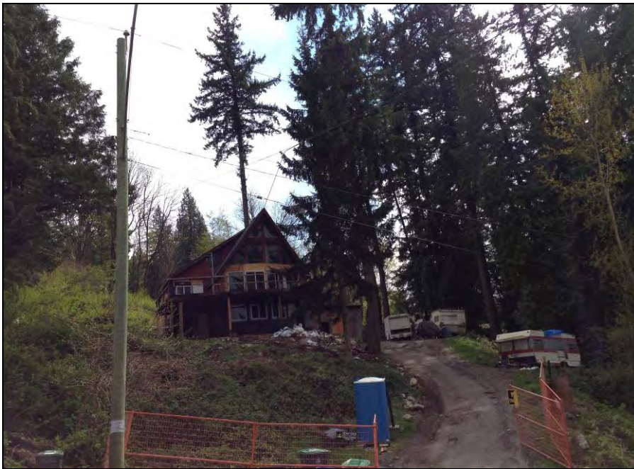
Photo 4: House under construction at 12512 Old Yale Road.
