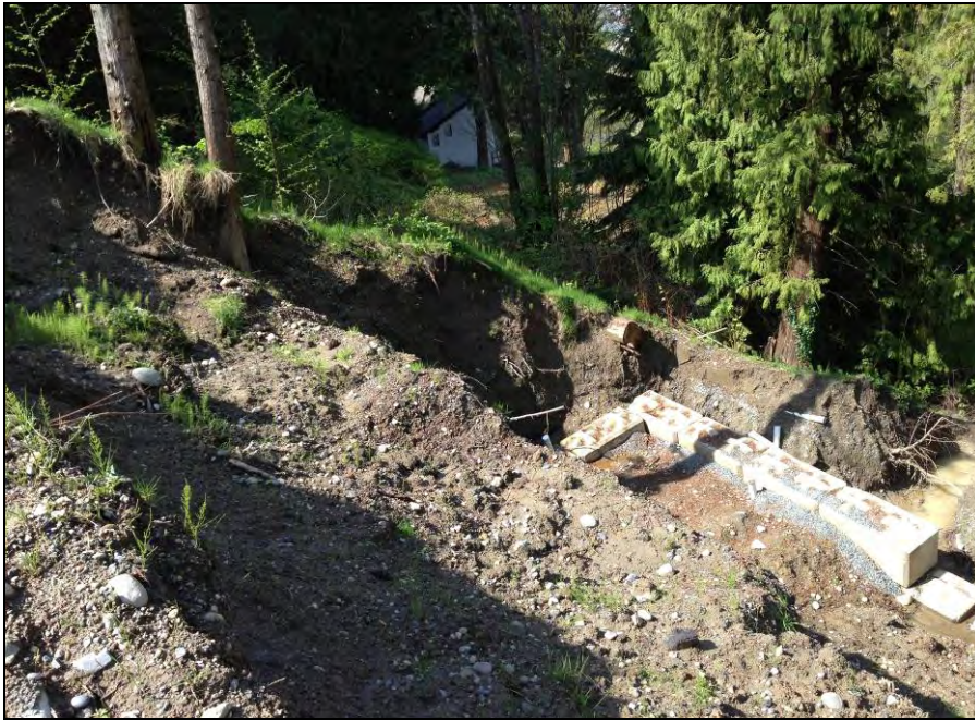
Photo 5: Excavations on steep slope for re-developments at 12701 – 107A Avenue.
