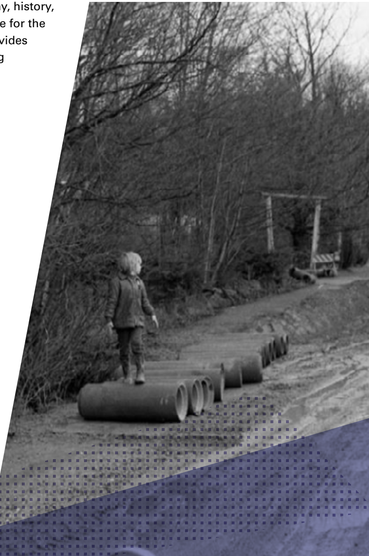
Above: Construction on 64 Avenue and 138 Street, Jan. 1974. Surrey Leader Collection.
