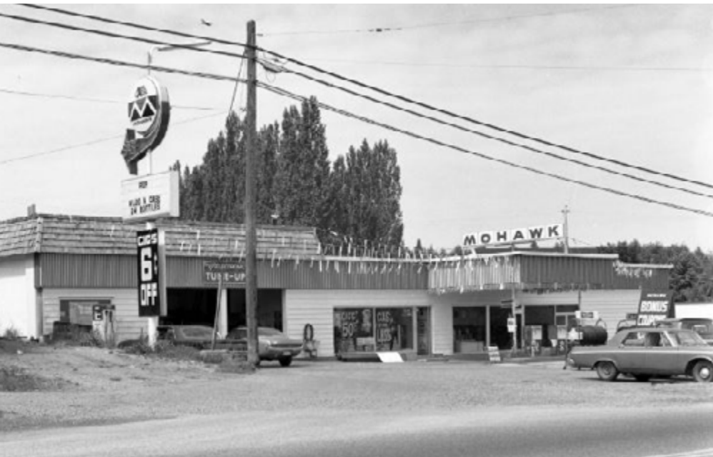
Above: Mohawk Gas Station located on located on the southwest corner of King George Highway and 62 Avenue, 1973. Surrey Leader Collection
