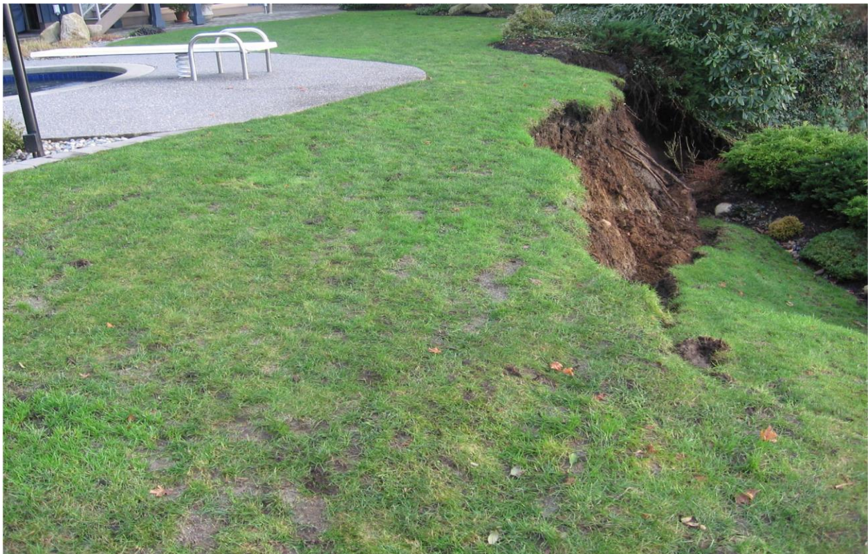
Unstable banks and steep slope hazards in Surrey.
