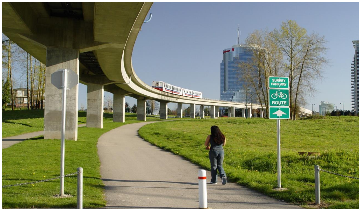
Multi-Use Surrey Parkway in City Centre, underneath the SkyTrain guide way.
