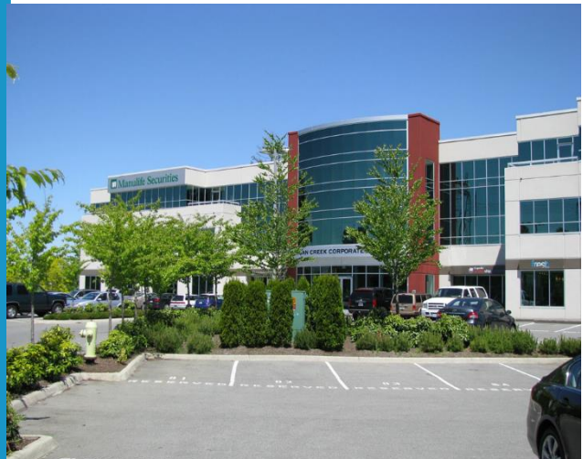
Example of Mixed Employment: Morgan Creek Business Park
