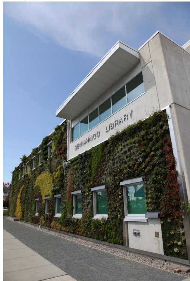
Living wall installed on Surrey's Semiahmoo
