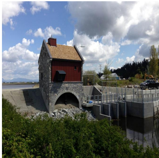
Crescent Beach pump station.
