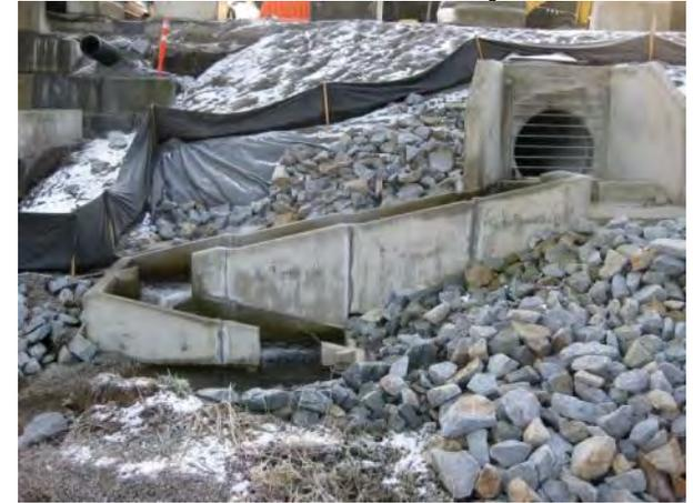
**Photo 30. Recently installed fish ladder installed during SFPR construction.**
