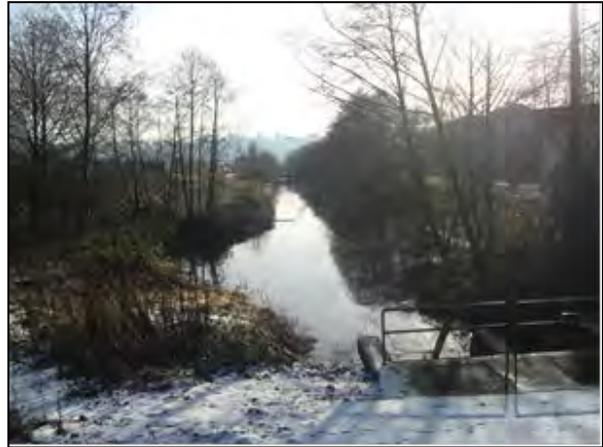
Manson Canal at Manson Pump Station. 11m width, 2.5 m height, 2H:1V Side Slopes
