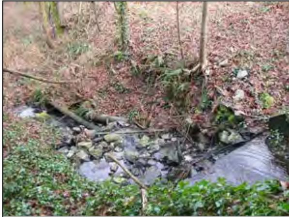
Scott Creek downstream of culvert at 99 Ave and Scott Road Diversion. Right bank showing signs of erosion.
