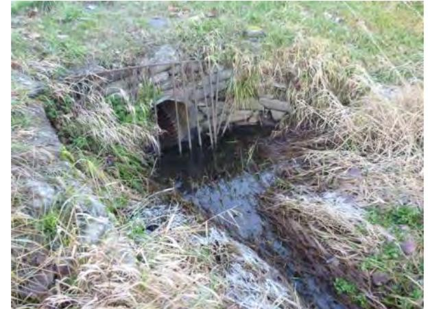
**Photo 18. Potential obstruction to fish movement.**
