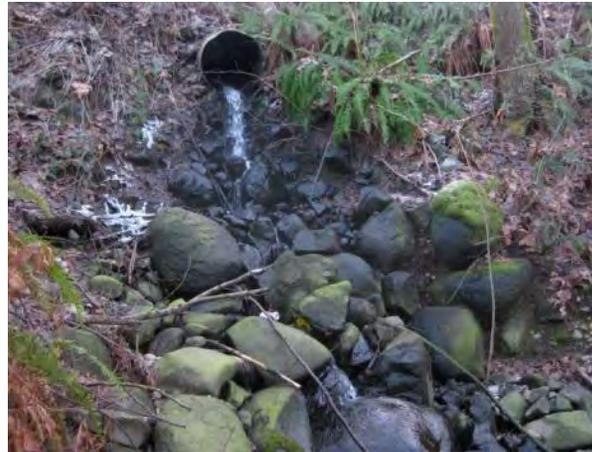
**Photo 26. Unstable Boulders – Shadow Creek culvert outlet at Queen's Place.**
