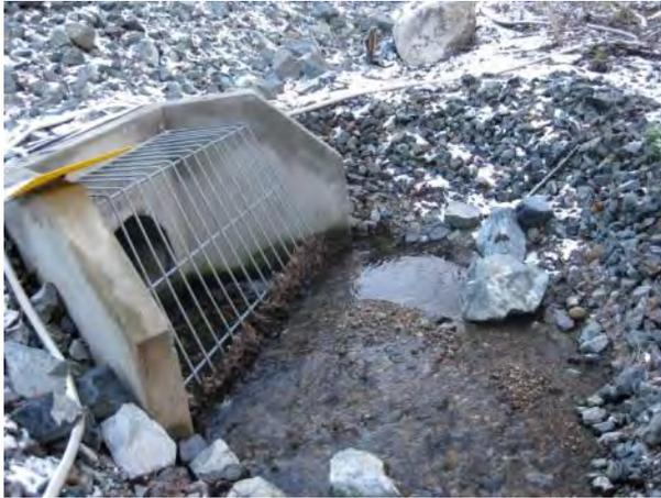
**Photo 28. New culver installed as part of SFPR construction.**
