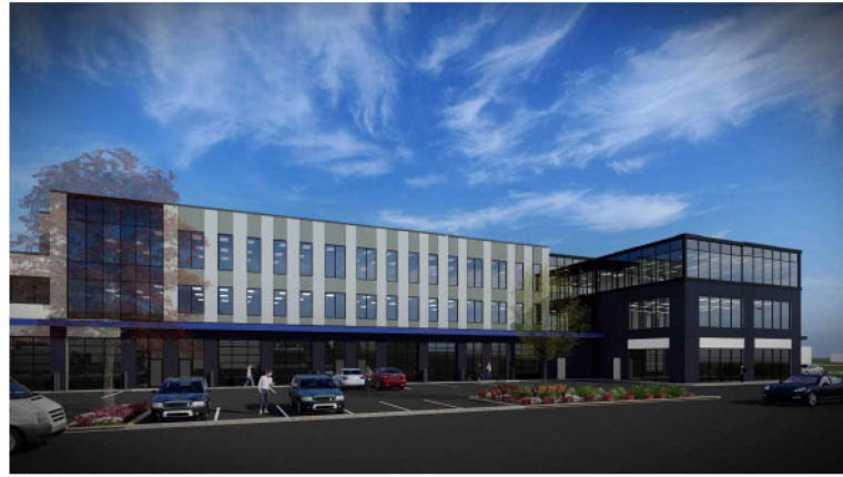
WEST VIEW OF OFFICES
